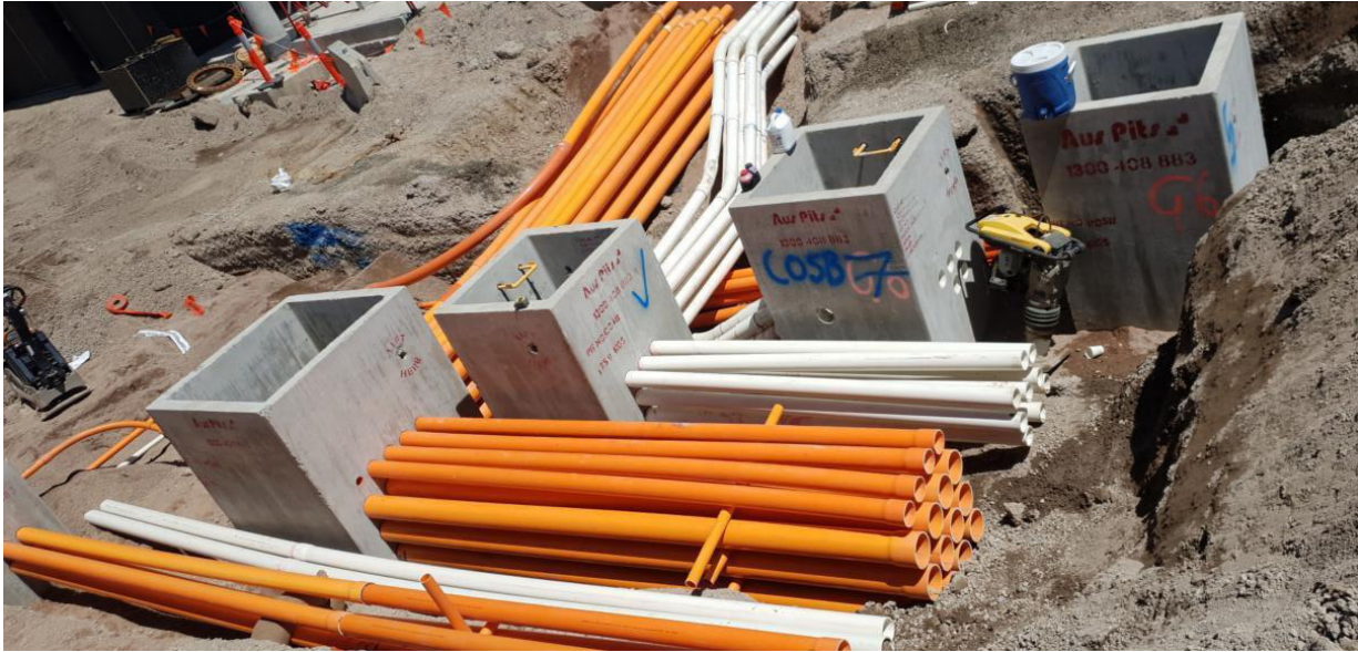
Westconnex M4 Widening - Stormwater installation, FRP and conduit installation
