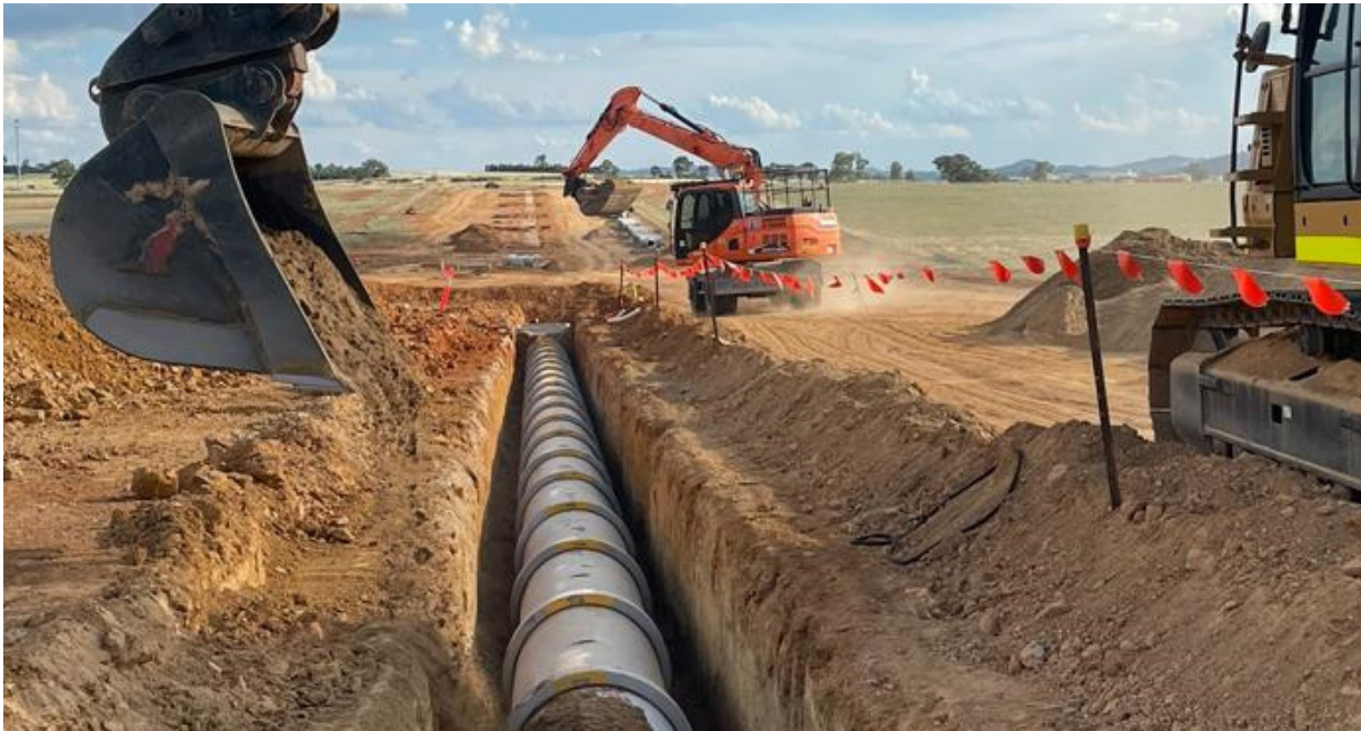
Wagawaga - Riverina intermodal freight and logistics hub - 5km of Stormwater RCP and FRC Pipe and Pit for Wagawaga council
